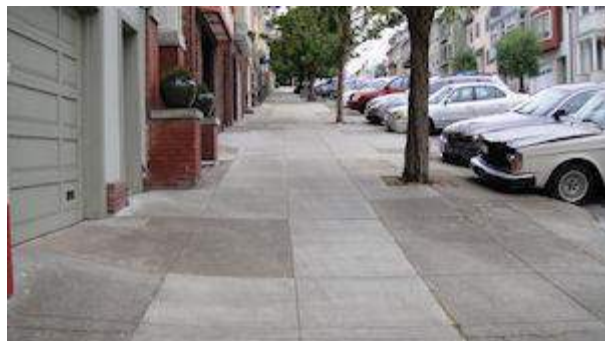
Figure 7 - 5th Ave. before Urban Watershed Stewardship Grant project
